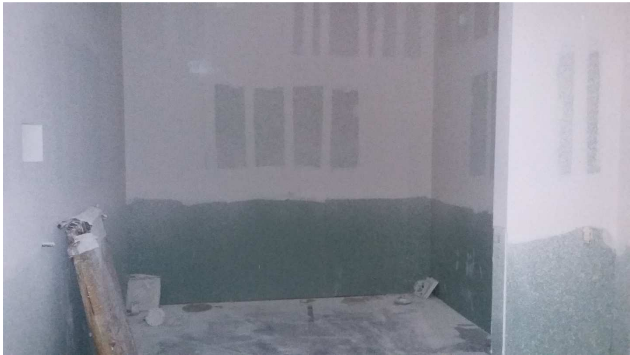
Interior view of the subject property (Unfinished Area)
