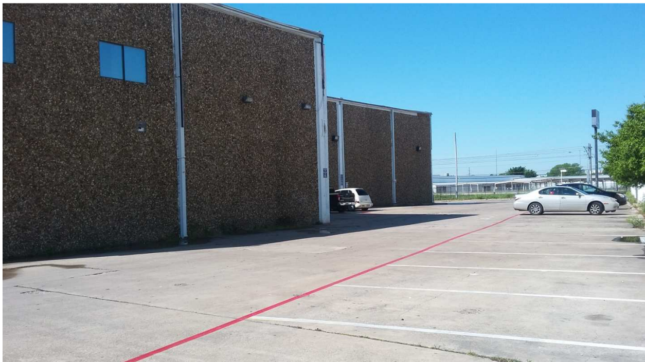
View of north elevation of the subject property
