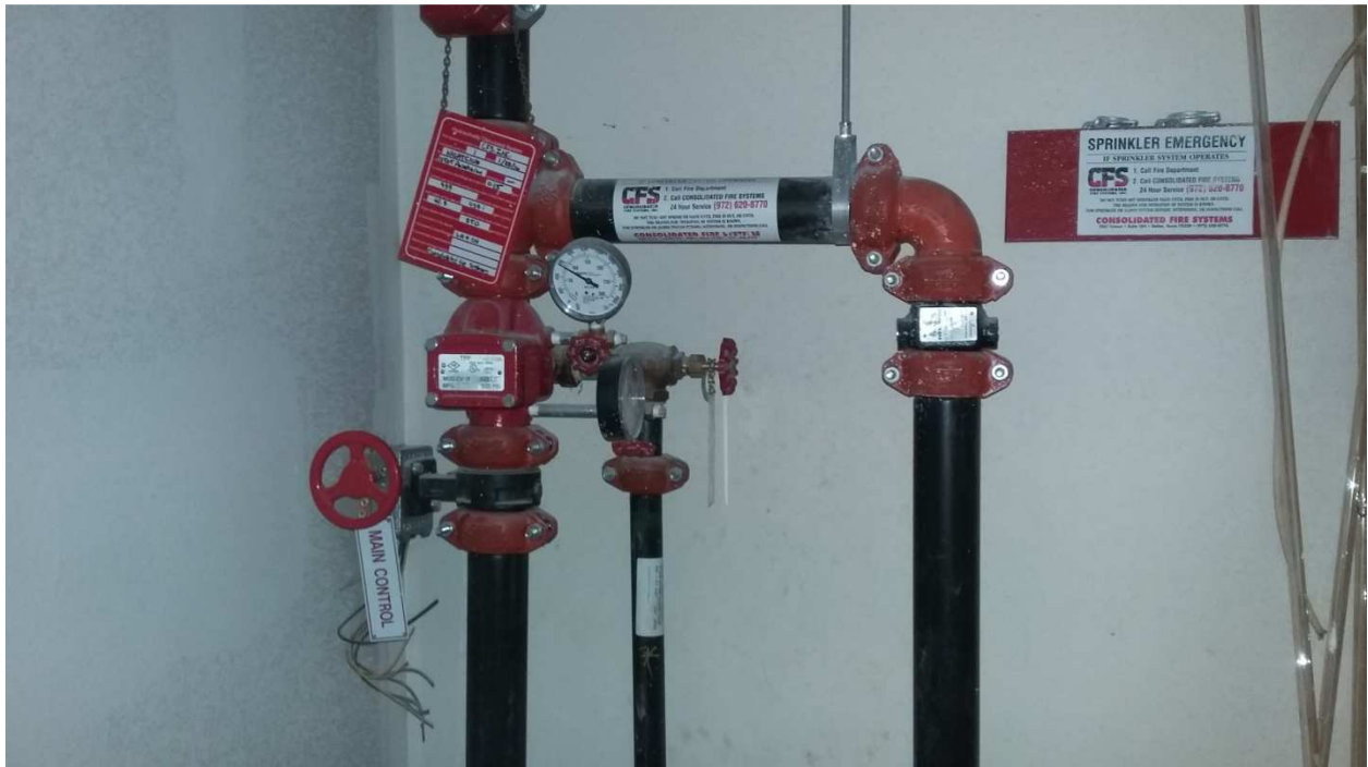
Interior view of the subject property
