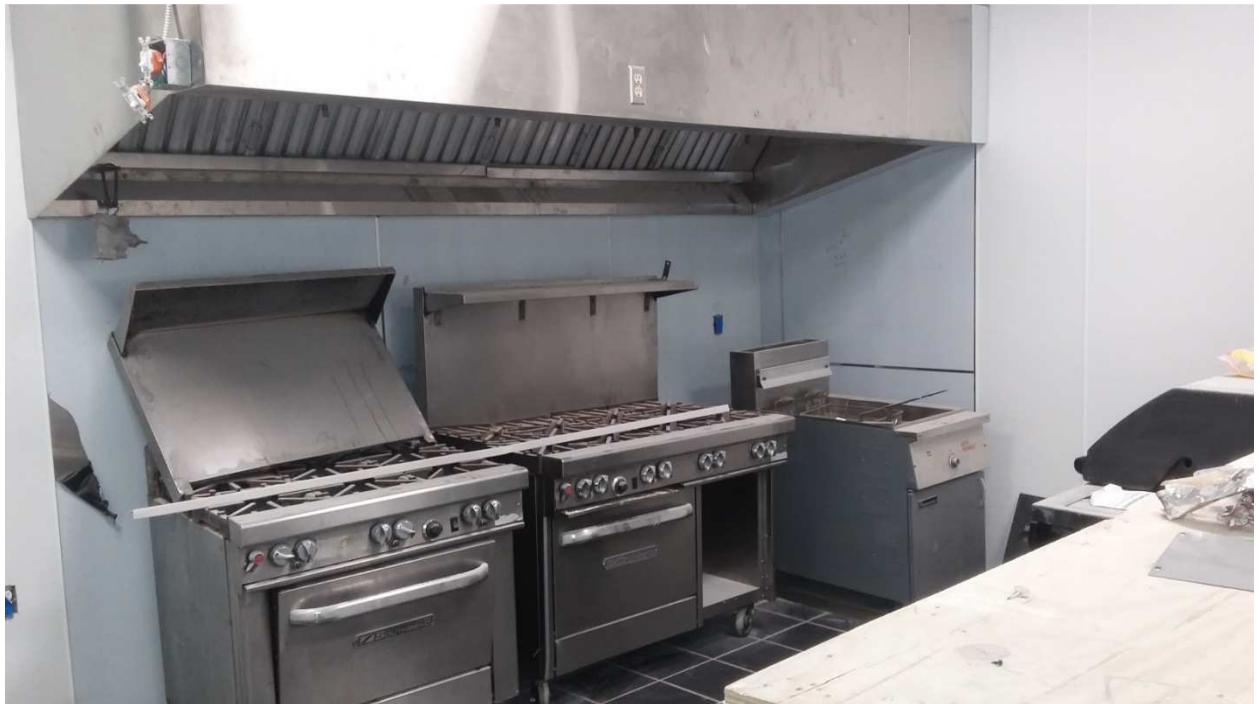
Interior view of the subject property (Kitchen Area)
