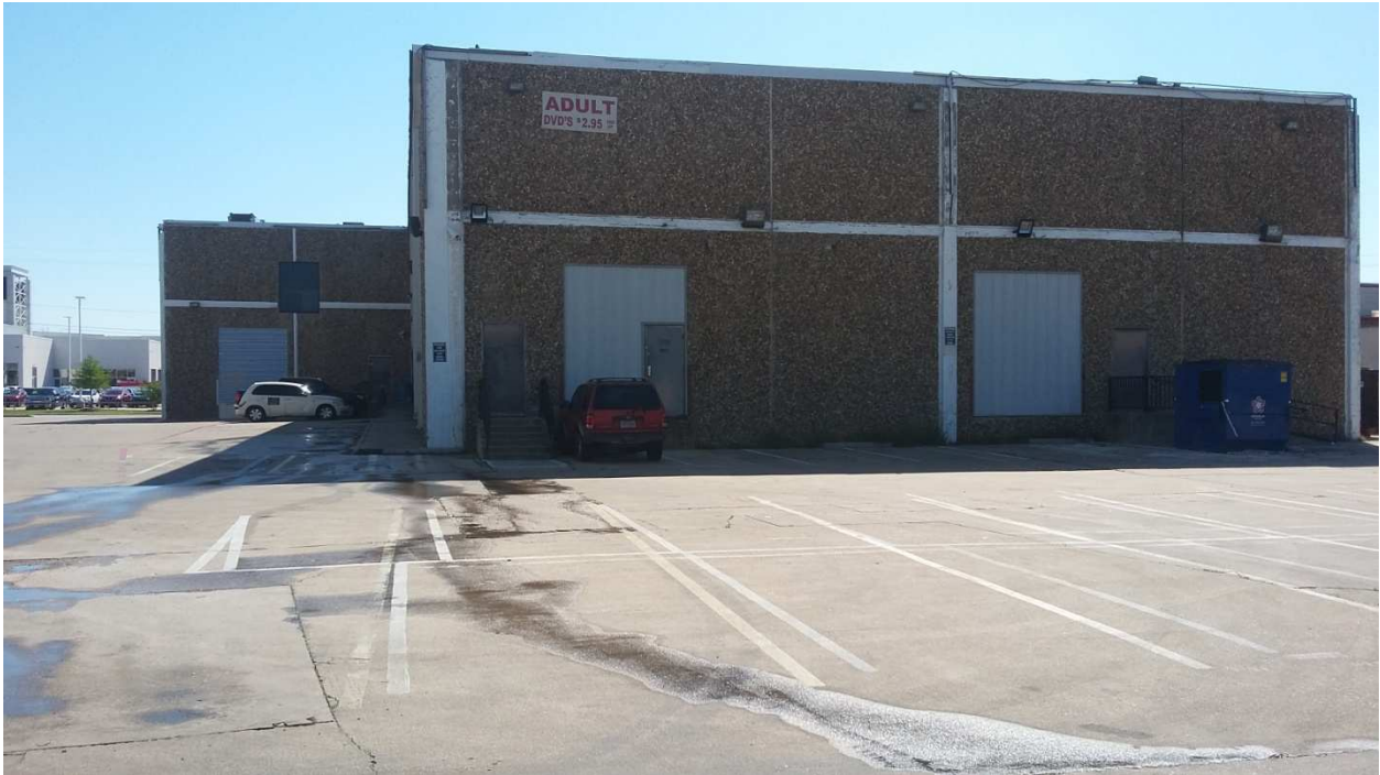
View of west elevation of the subject property
